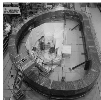
Fig.2 3 rd TF coil WP after impregnation
