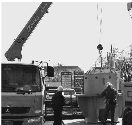
Fig.1 Installation of Mobile Pilot plant
