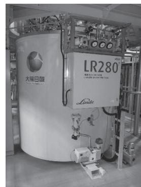
Fig.1 Photograph of 600 W variable temperature helium refrigerator/liquefier in NIFS.
