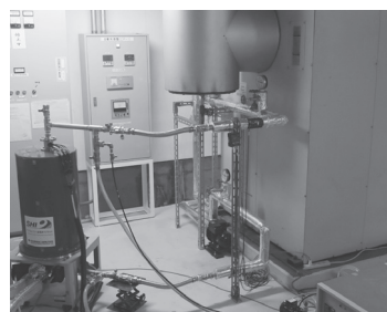
Fig.1 HGMS system introduced to the heater boiler system in a factory.
