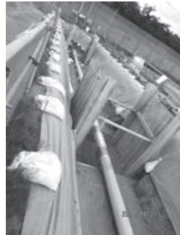
Fig.1 Installation of cryopipe.
