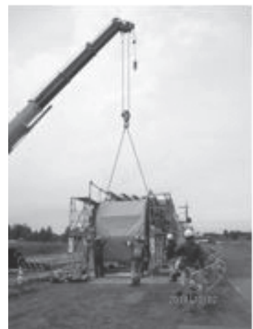
Fig.2 Preparing for cable core installation
