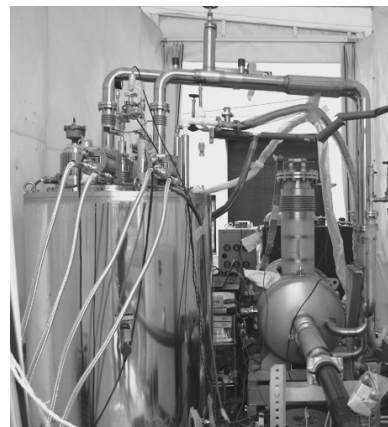
Fig.3 Photograph of cooling system for 30-m superconducting cables
