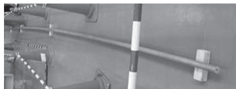
Fig. 4 Blasted conductor after the straighten process.
